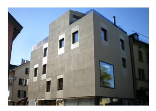
The Wohnhaus/Residence project entailed the design of a combination ofreinforced concrete flat slabs, shear walls and columns as structural system. The irregularity of the building, both in plan and elevation, posed a designchallenge. However, a careful modeling of the structure was undertakenusing SOFiSTiK. Ultimate Limit State and Serviceability Limit States were checked for various load combinations including earthquake action.
